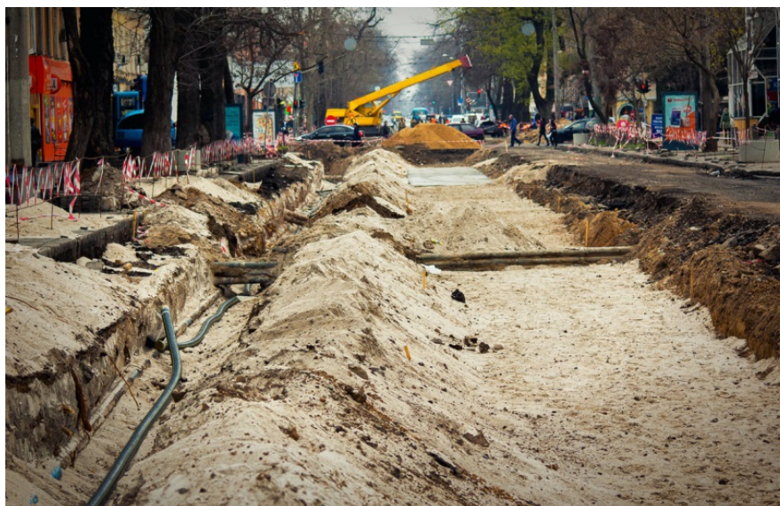
Pic. 8. «Replacement of engineering networks near the "Passage"»
